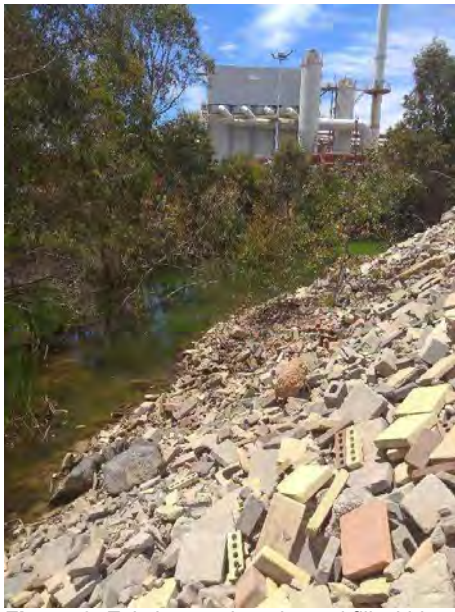
Figure 6: Existing earthworks and fill within application area
