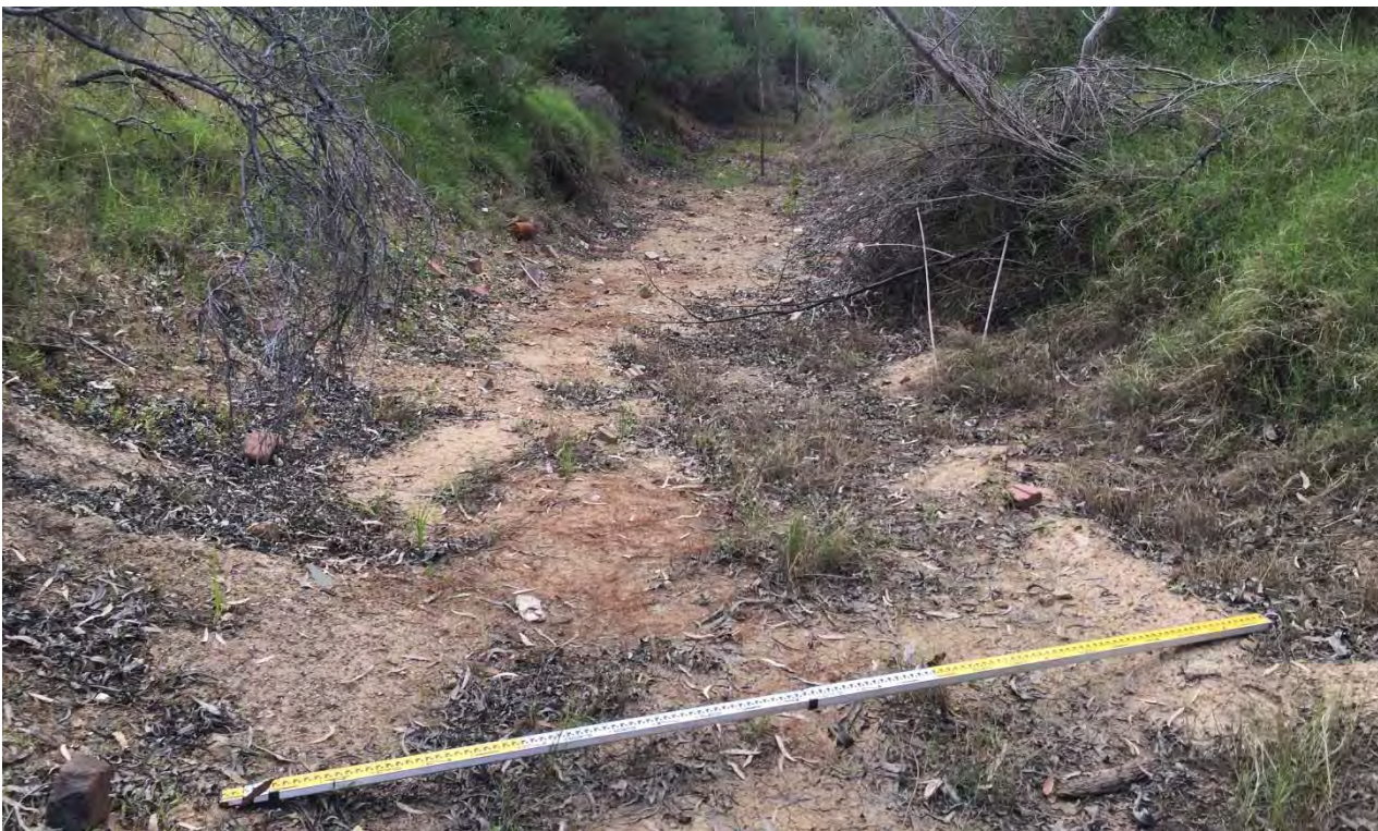
PLATE 20: Open drain from southern storage areas to southern outlet
