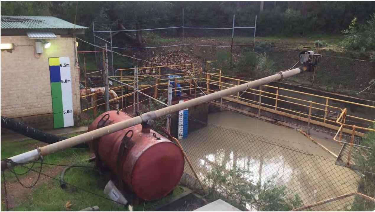
PLATE 9: Main Site Sump and Pump. Main Electric Pump (170 l/s) located in building
