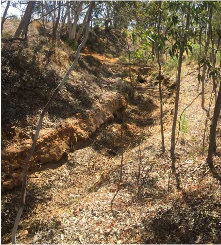
PLATE 17: Existing open drain along western boundary to convey water to southern storages
